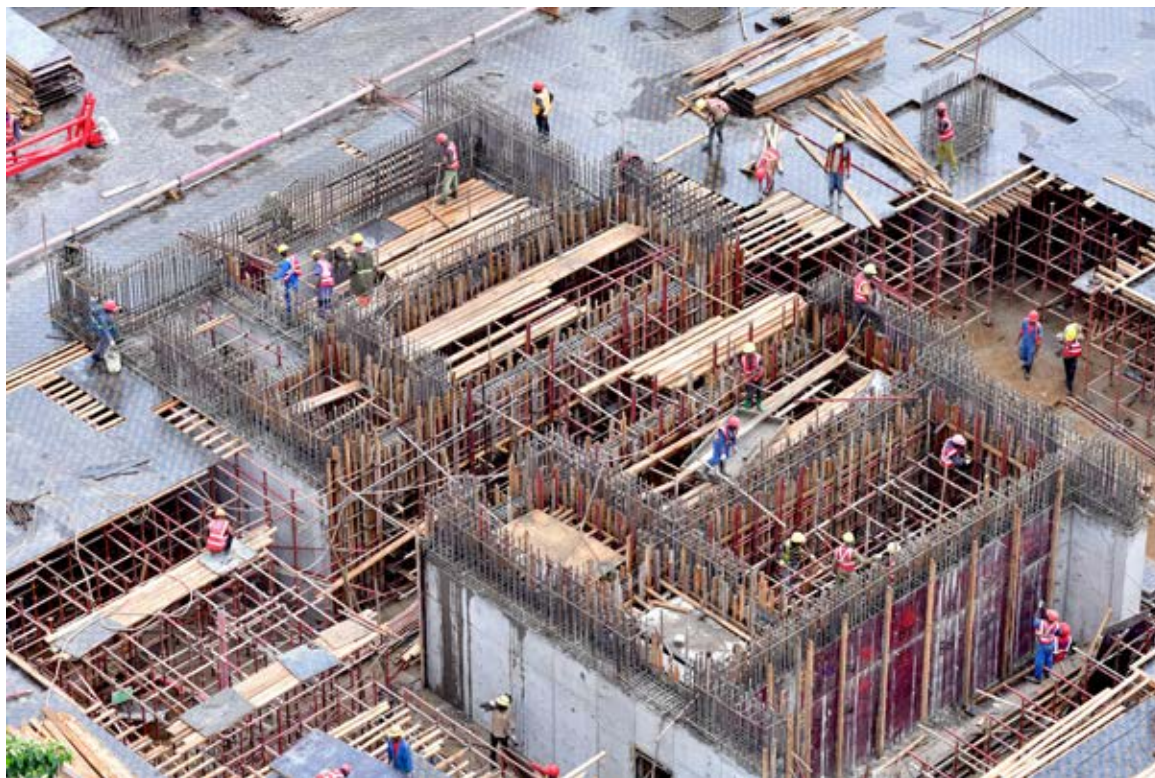
Development needs investment: Major construction site in the Rwandan capital Kigali.
