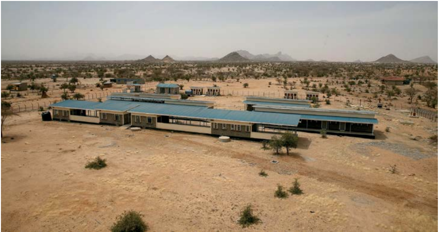
As a result of decentralisation, hospitals are now also being built in Kenya's desert regions.
