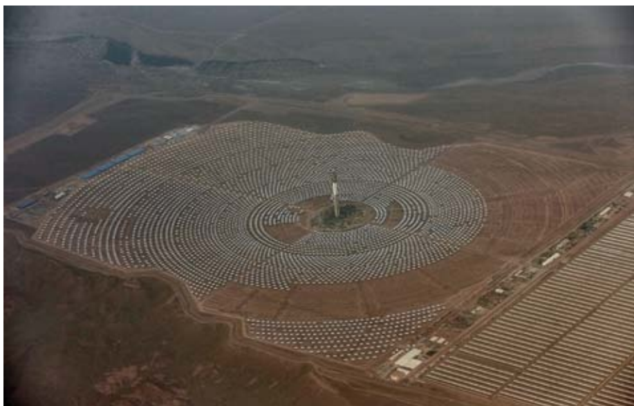
German ODA supported the solar power plant Noor 3 in Ouarzazate, Morocco.
