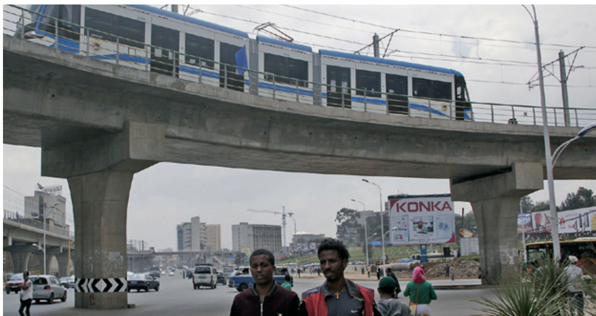
China supports building African infrastructure: the light rail in Addis Ababa is an example.
