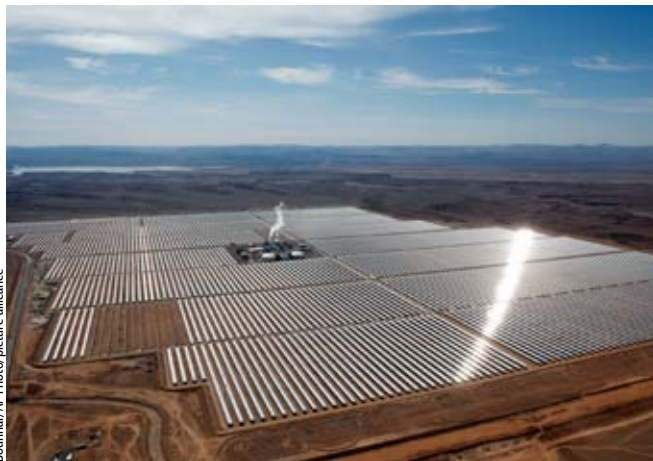
The world’s largest concentrated solar power plant is located in Ouarzazate, Morocco.
